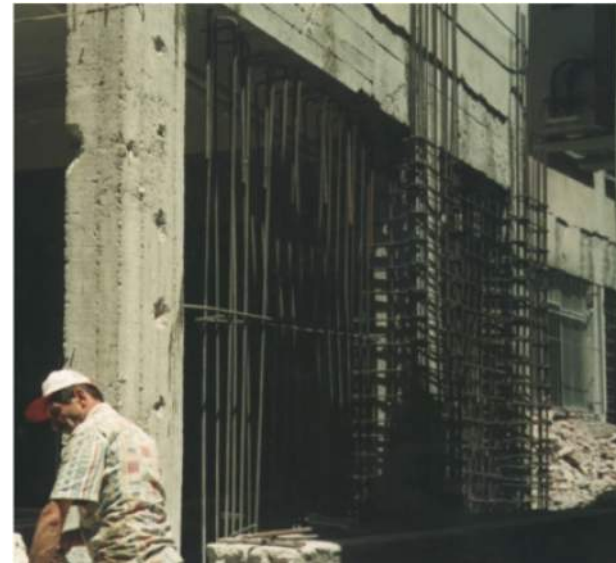
Shear wall strengthening, Bolu, 2000
