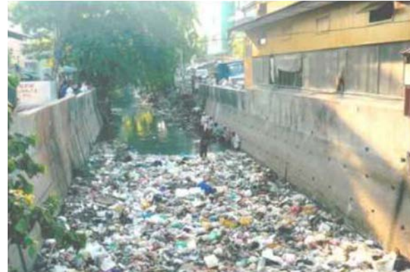
Solid waste accumulation obstructing the drainage system
