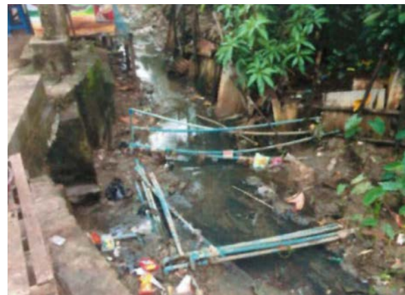
Utility pipes obstructing the flow and increasing the amount of stuck objects
