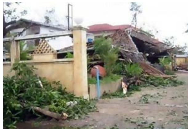
FIGURE 25. Residence damage due to Cyclone Nargis in Yangon (MES, 2017)
