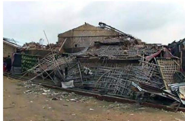
FIGURE 27. Residence damage due to Cyclone Mora in Sittwe (RFA, 2017)
