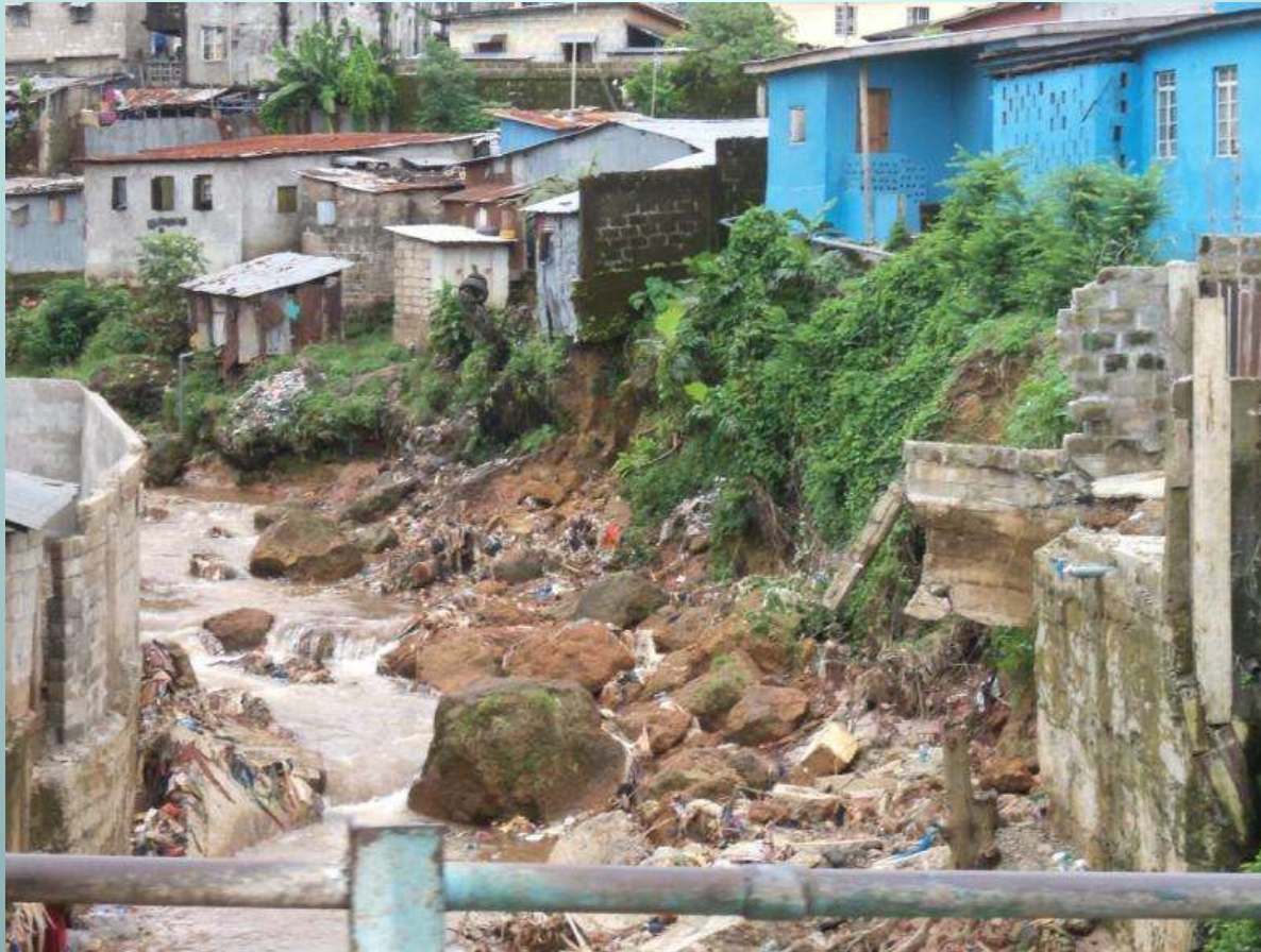
Erosion of Stream Bank, Savage Street Bridge
