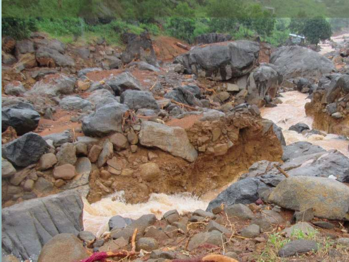
Erosion along stream bed – Regent landslide area
