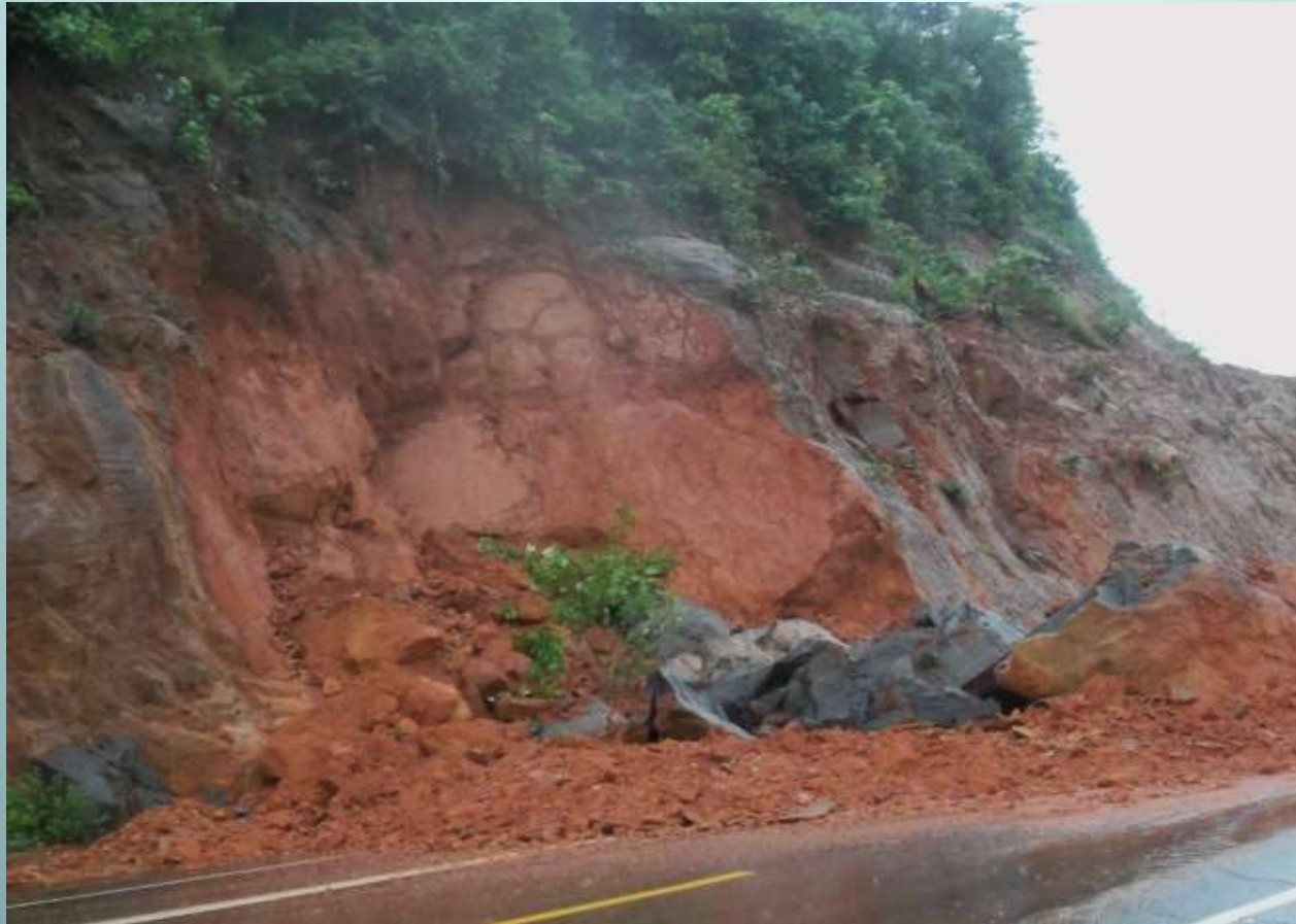
Slope failure and Rock fall (September 2016) along the Regent - Grafton road (Bathurst village)
