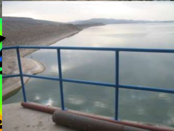
Irrigation dam with over 100,000 people at risk (downstream)
